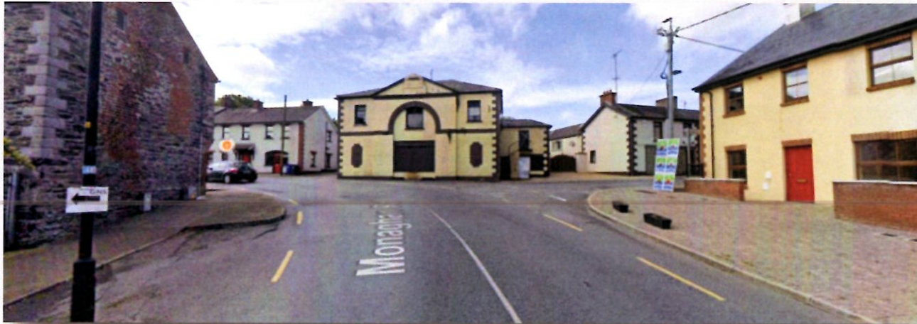
Existing Street View – Poorly presented streetscape / vacancy, expansive roadway and vehicular priority
