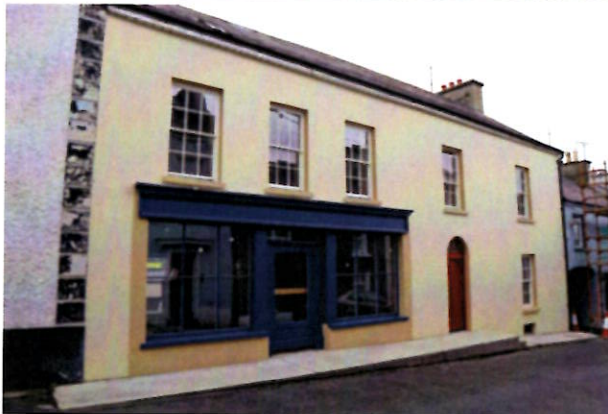
Ramelton Co Donegal —Adaptation and Reuse of historic dwelling, reinstatement of shopfronts, and reinstatement of lime render by Dedalus Architects Illustration of before and after
